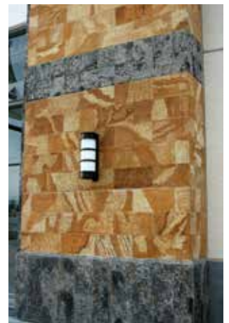
A multitude of stone appearances were created from architectural precast concrete to add a distinctive style to the massive Paseo Altozano (Altozano Walkway) shopping center in Morelia, Michoacan, Mexico. Rubber molds made from actual stones, including slate, ensured the accuracy of the precast concrete appearances. A variety of finishes added texture.
