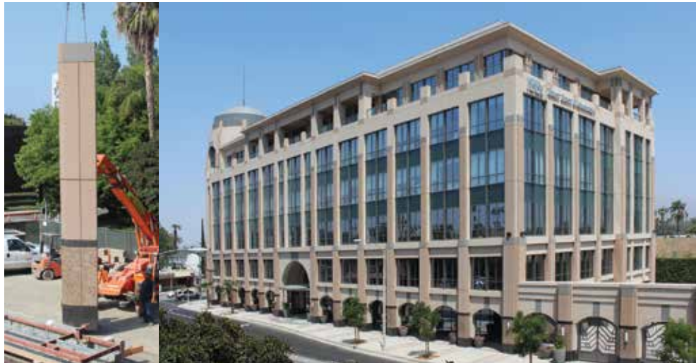
Citrus Tower Corporate Plaza sets a new standard for aesthetic design in Riverside, Calif. It features GFRC panels on its façade in three colors. GFRC was chosen because of its ability to create the complex appearance desired, including multiple colors in one panel. Its light weight saved on framing costs and made the pieces easier to handle.
